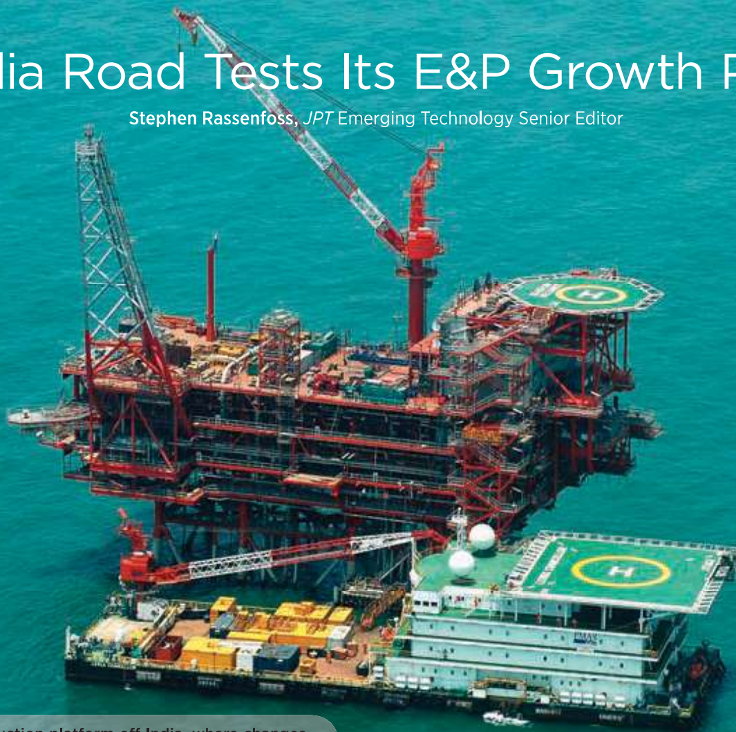
A BP production platform off India, where changes in the rules are designed to revive exploration and production activity by international oil companies. Source: BP.
